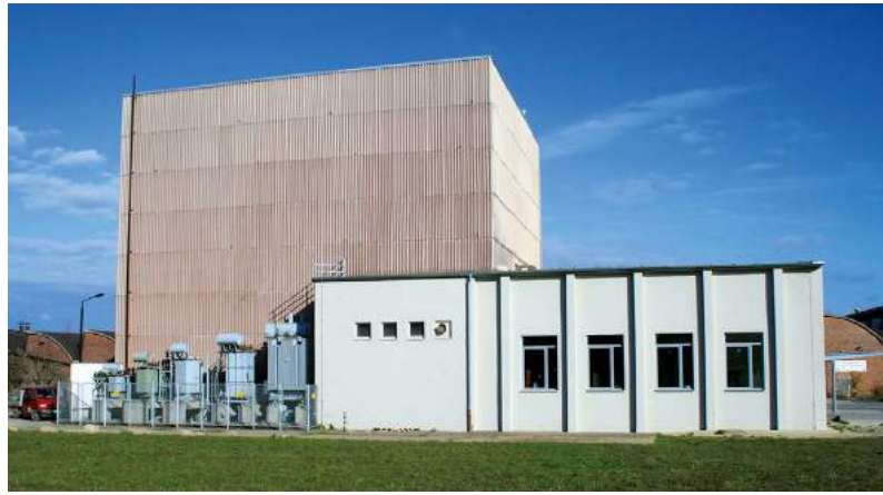
Test lab | Hermsdorf / GERMANY
